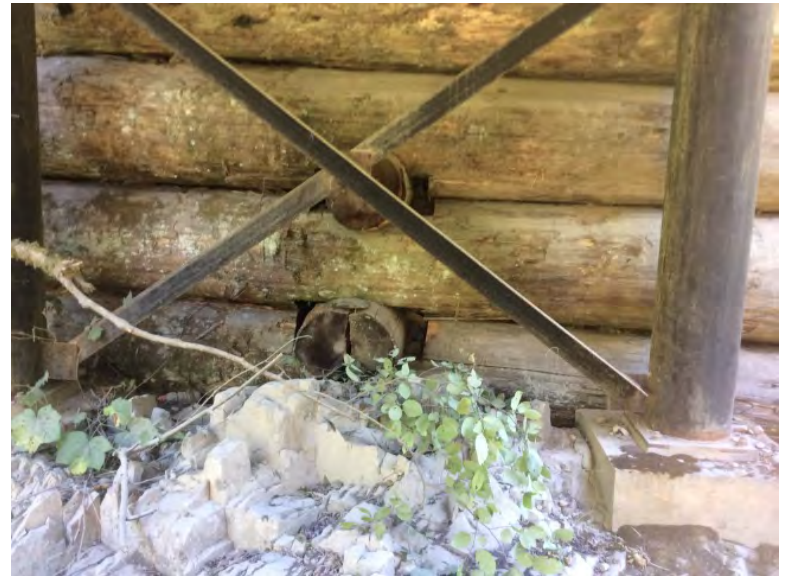
Right Bank Abutment when facing downstream
