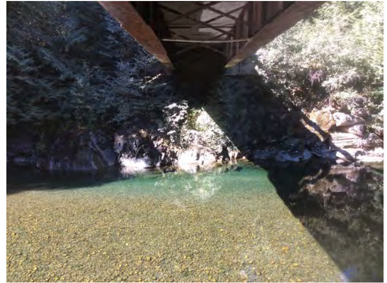
Left Bank Abutment when facing downstream
