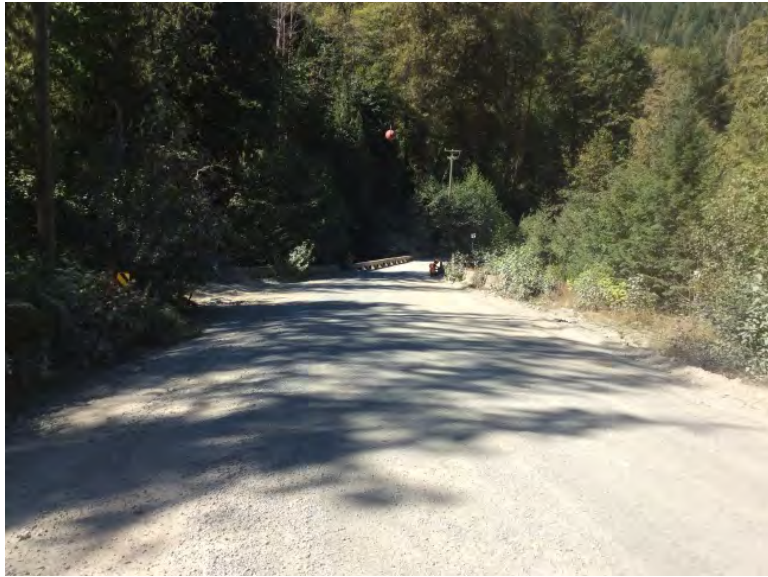
Approach from Right Bank when facing downstream
