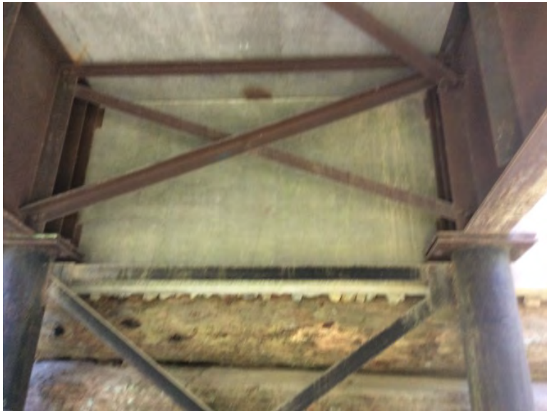
Right Bank Abutment when facing downstream
